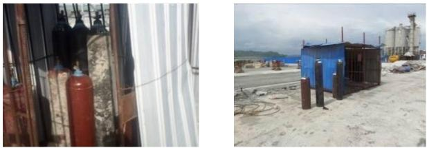
Figure 5.1 Examples of Near Misses - Gas cylinders incorrectly stored and handled
